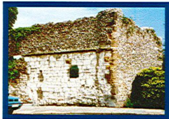
Blackfriars Priory, Arundel Chalk
